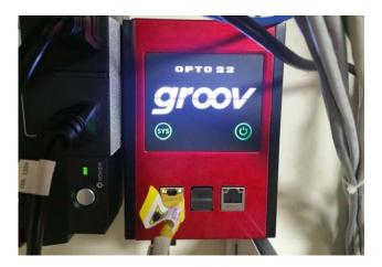
The SNAP-PAC-R2 controller pulled data in from a variety of Modbus devices. Once the Modbus data points were in the SNAP PAC, the *groov* appliance allowed Bravo to quickly build mobile screens to monitor Freon<sup>™</sup> detection sensors, cold room temperatures, compressors, and even the factory's condenser tower.
