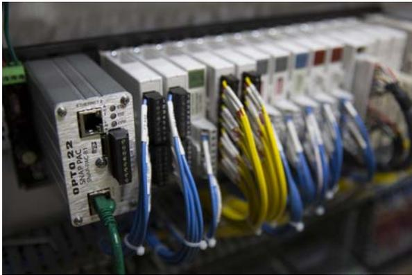
*Opto 22 PAC controllers and SNAP I/O modules are used to monitor and control all processes.*
