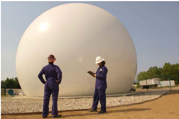
Methane collected in a giant balloon is transported to the New Belgium facility and used as fuel
